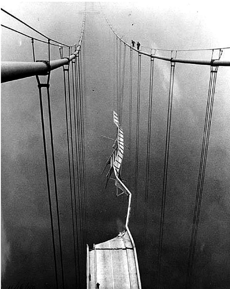
Most Tacoma Narrows / Tacoma Narrows Bridge (1940)
